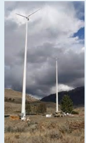
Wind Turbines at the new Nighthawk POE
