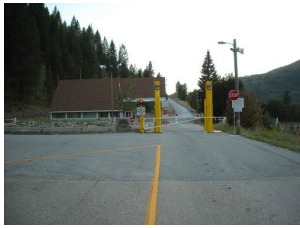
Recently de-commissioned Boundary POE
